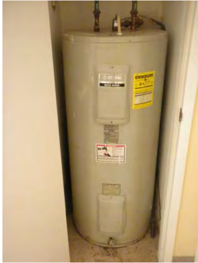
Example of an electric domestic hot water tank
