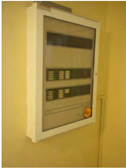
Central Fire Alarm Control panel
